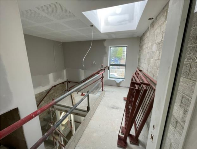
Balustrading installation to Preedy under way
