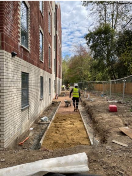
Hard landscaping behind MacDonald underway
