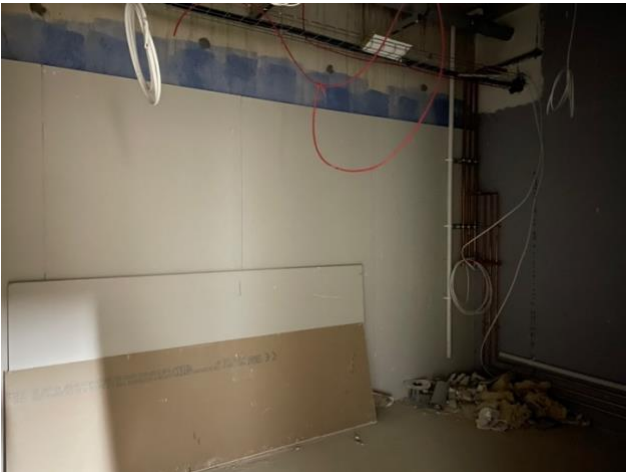
Laundry room in the basement of Townsend in progress
