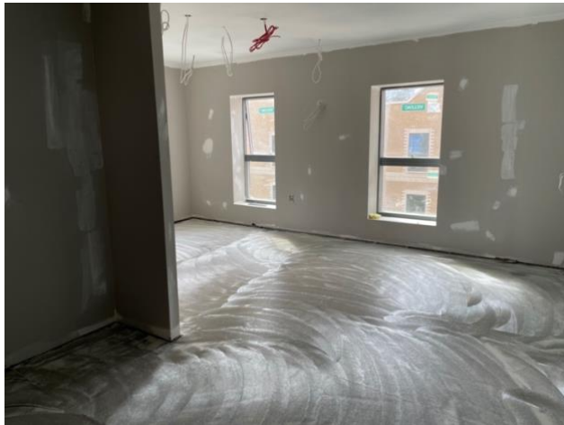
Flooring in progress
