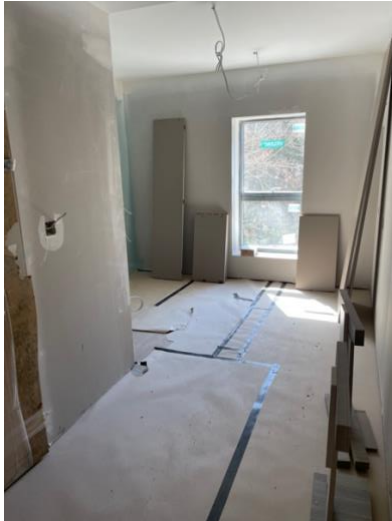
Furniture installation in progress on Beddoe's ground floor
