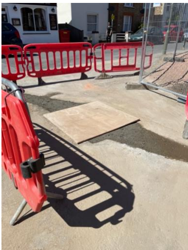
Manhole completed in entrance
