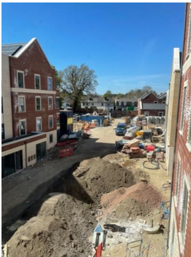
Site court yard 23 April
