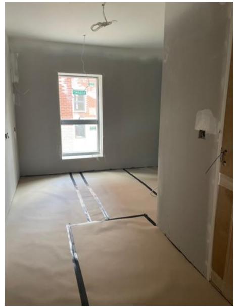
Mist coat applied to 2nd floor corridor in Townsend. Cluster bedroom in Townsend with mist coat – 1st floor
