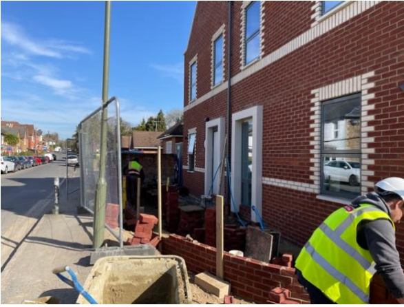
External wall in front of Parfitt being installed
