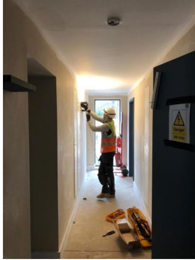
Wall lights being fitted in corridors
