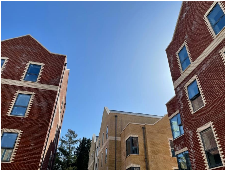
Townsend, Beddoe and MacDonald all completed externally
