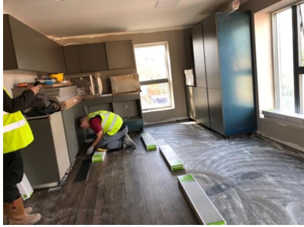
Floor to cluster kitchen installation underway
