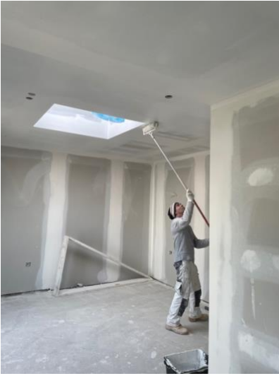
First coat to 3rd floor of Townsend
