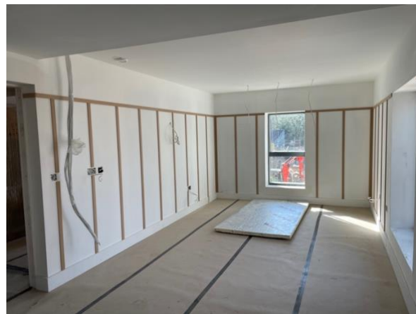
2nd fix carpentry cluster kitchen in Preedy ready for decoration
