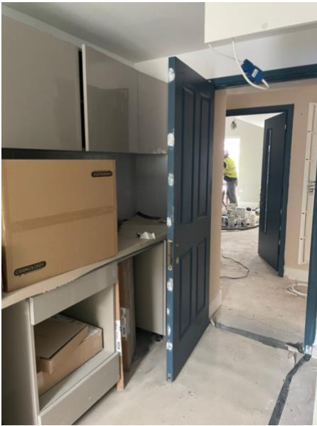
Entrance doors installed with 1st blue coat.
