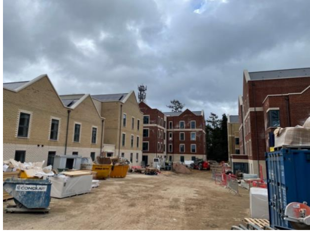
Site view with no crane!
