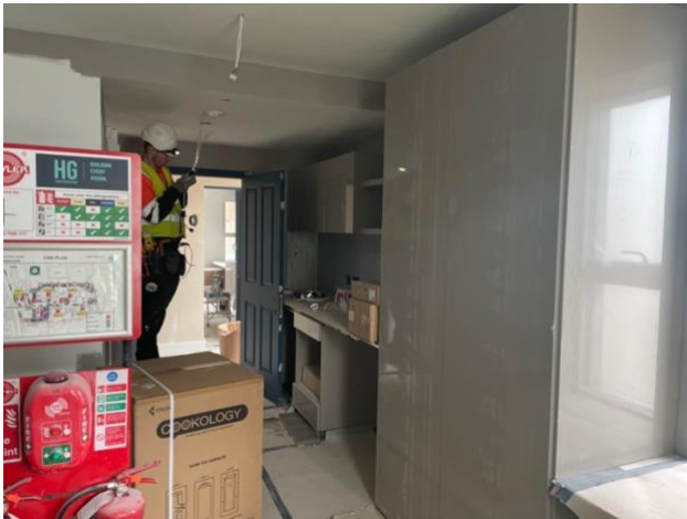
Final electric works to Parfitt underway
