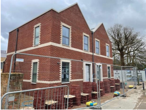
External works to Parfitt underway on Harvest Road
