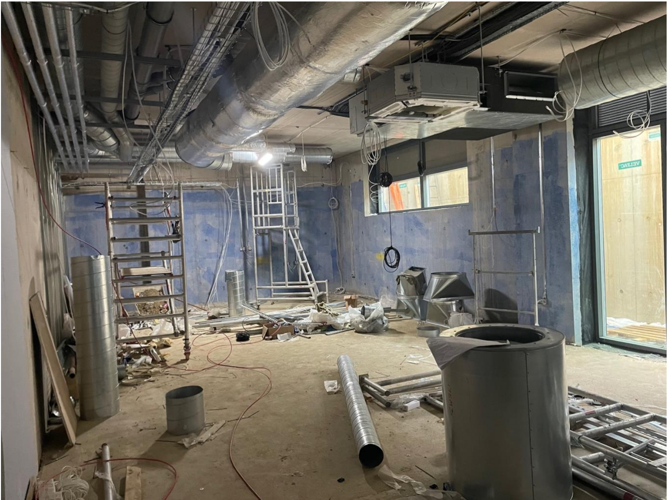
Basement communal room – getting ready for plasterboard ceilings coming week
