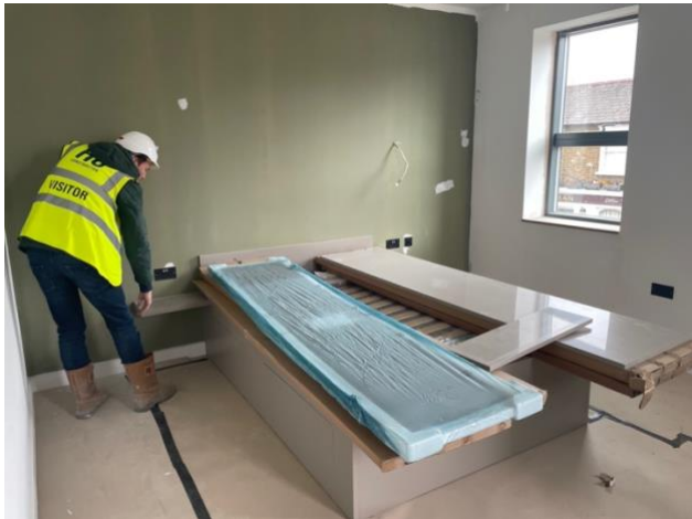
Furniture installation underway in Parfitt
