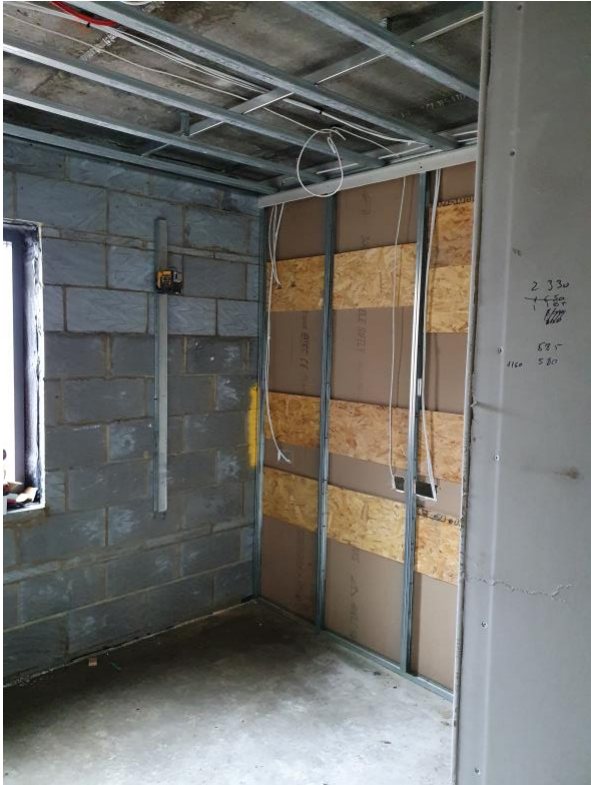
Metal stud work and electric 1st fix to Preedy 1st floor
