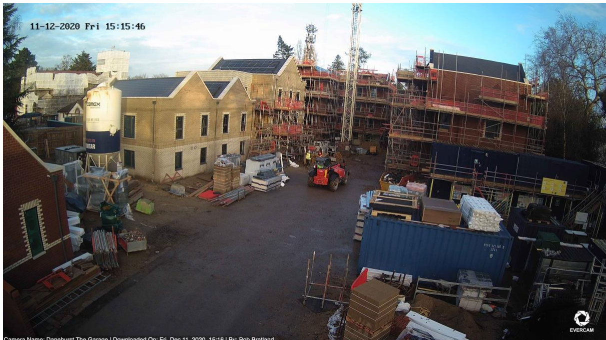
Preedy with almost no scaffolding!
