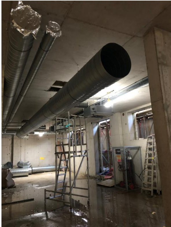
Ventilation system installation to basement of Townsend
