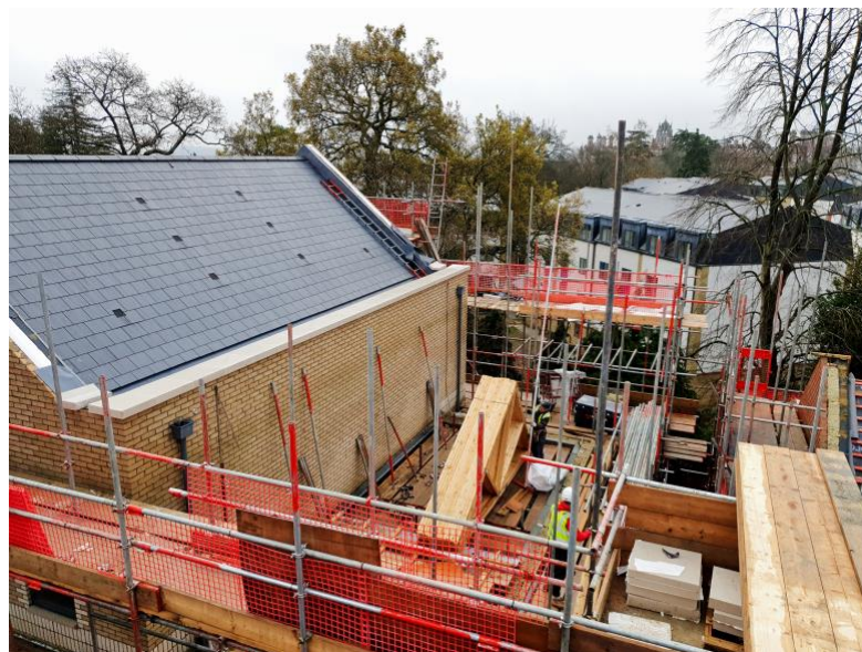
Low level roof trusses to Beddoe
