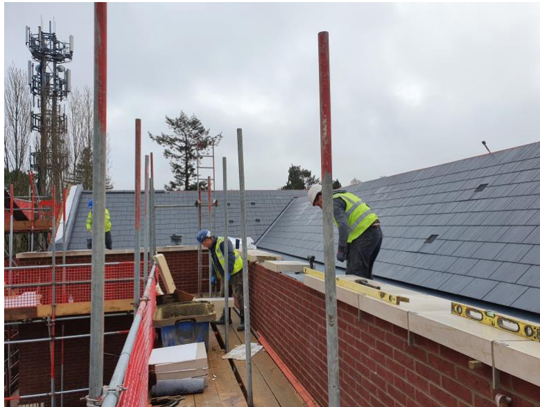
Coping installed to roof on Townsend
