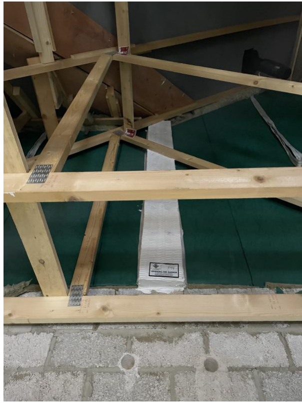
Fire stopping installed in joints to roof space
