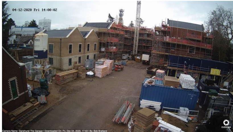
½ of Preedy without scaffolding
