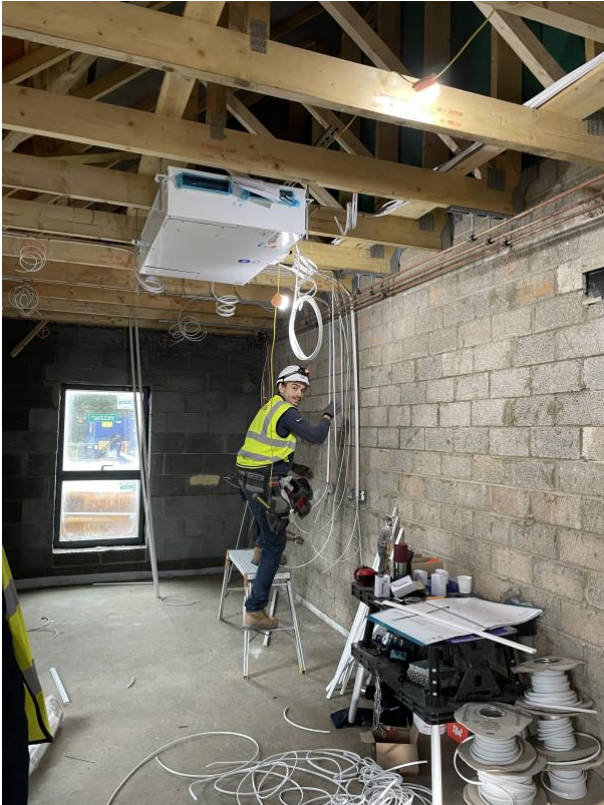
Electric 1st fix in progress in Preedy
