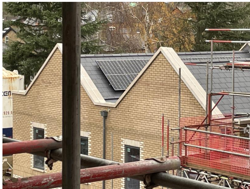
Solar panels on Preedy's roof installed
