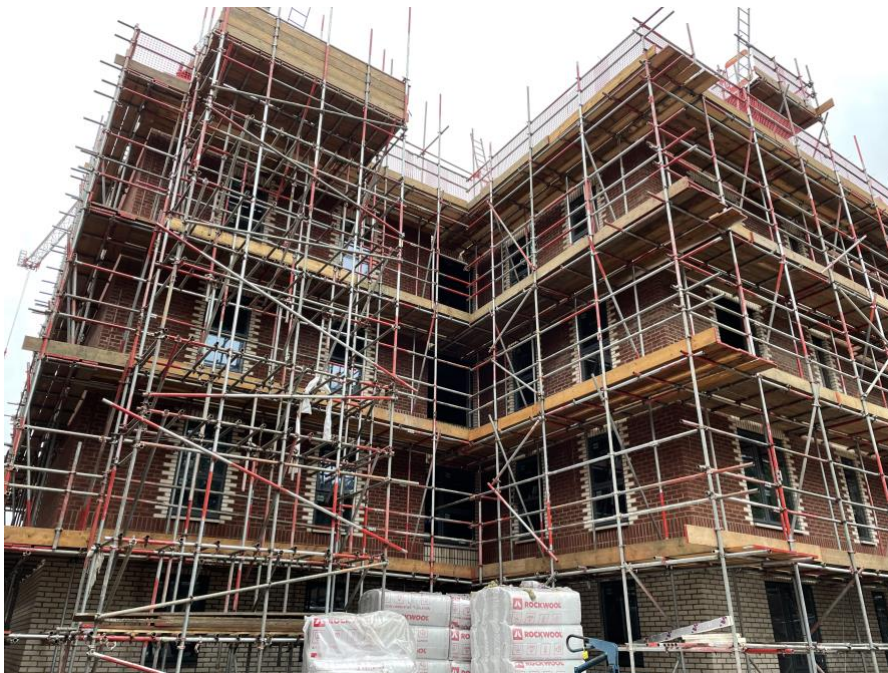
Townsend still surrounded by scaffold
