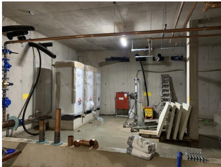
Plant room installation has started
