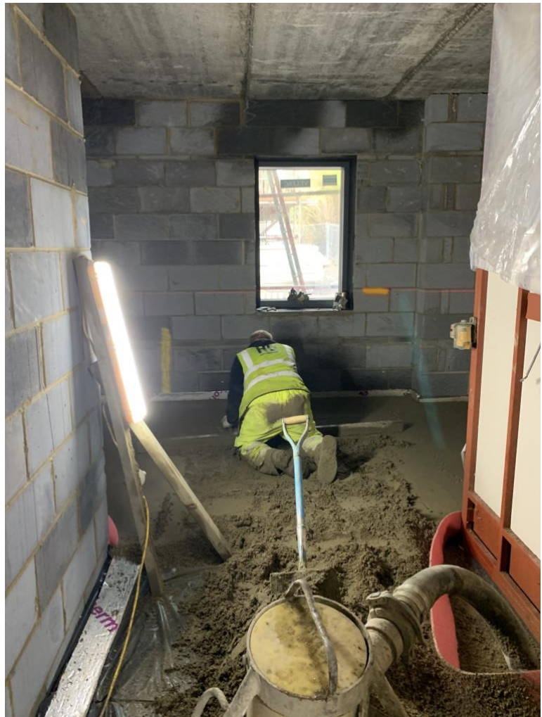
Screeding underway to ground floor of Beddoe 13.11.2020
