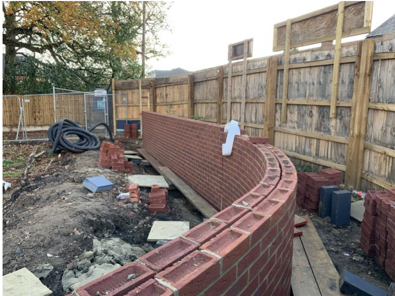
Brick wall facing Harvest Road under construction
