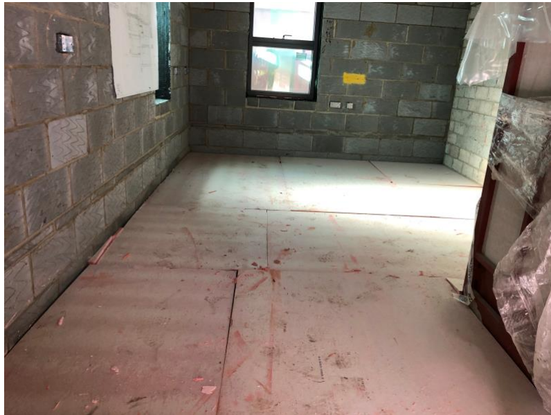
Insulation installed prior to screeding in Parfitt
