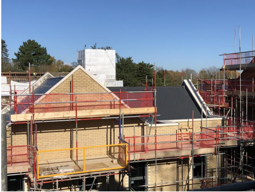
Roof works to Preedy complete
