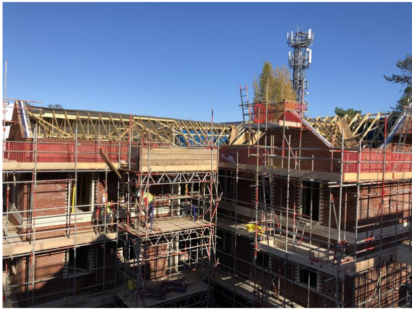
Carpentry works to Townsend complete for felt and batten to start
