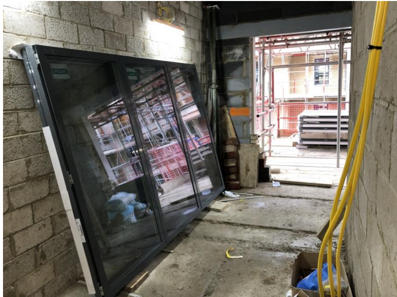
Entrance door set for reception in MacDonald has arrived
