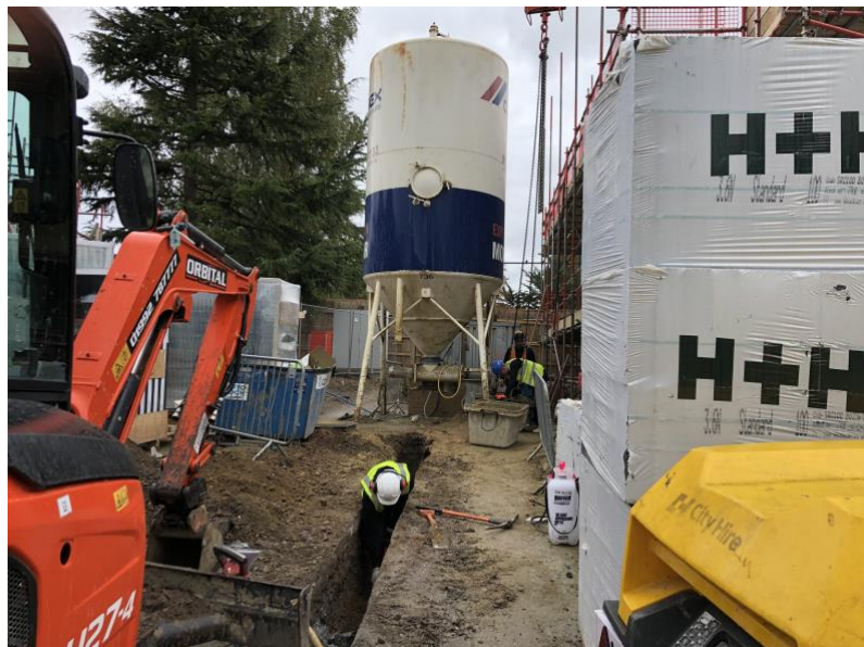
Trench being prepared for gas connection
