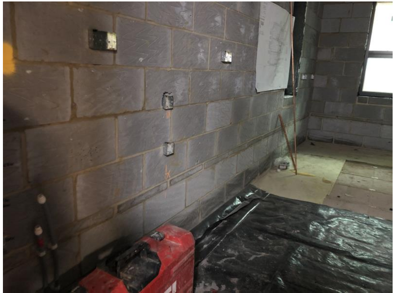
Electrical first fix in progress
