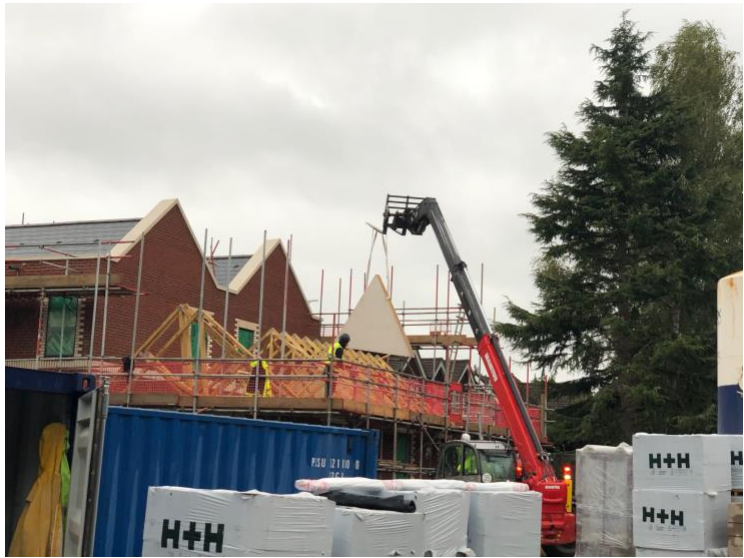
Parfitt with upper floor complete with coping and windows installed
