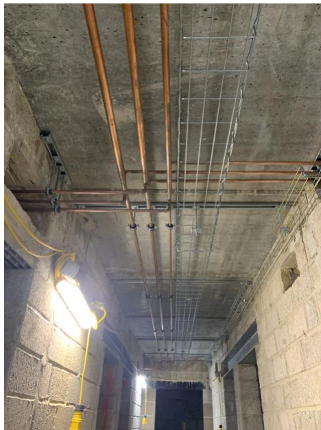
Plumbing progressing in Preedy
