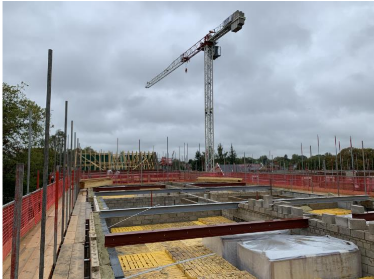
Roof level of Beddoe looking towards MacDonald
