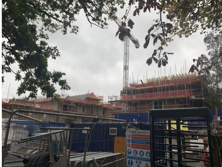
Progress seen from the pedestrian entrance
