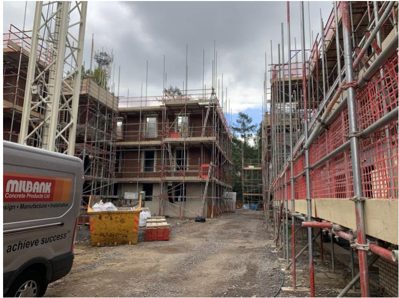
View of internal courtyard
