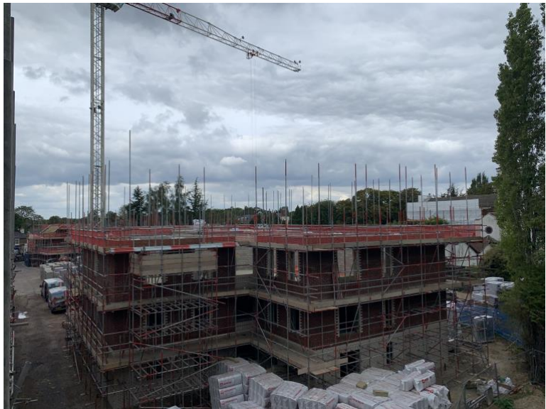
View of Townsend at 3rd floor level
