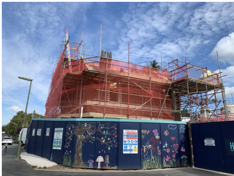
Parfitt roof being installed
