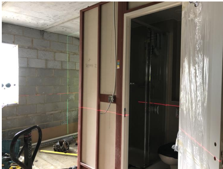
Setting out of the first shower Pod install
