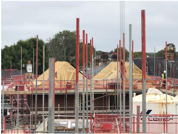
Parfitt seen with roof trusses now installed
