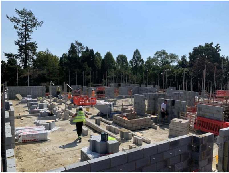
MacDonald progressing towards 3rd floor following slab installation
