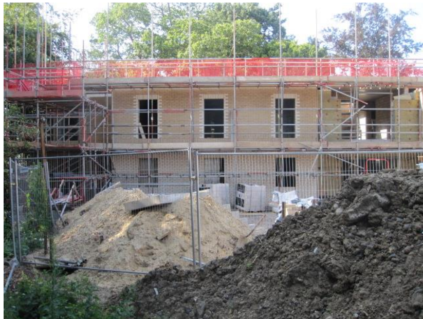
East elevation of Beddoe taking shape
