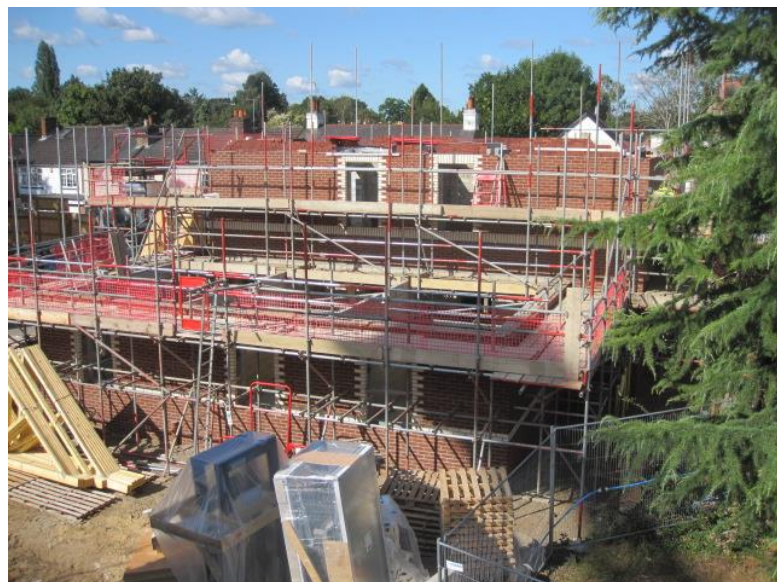
Parfitt 1st floor almost completed
