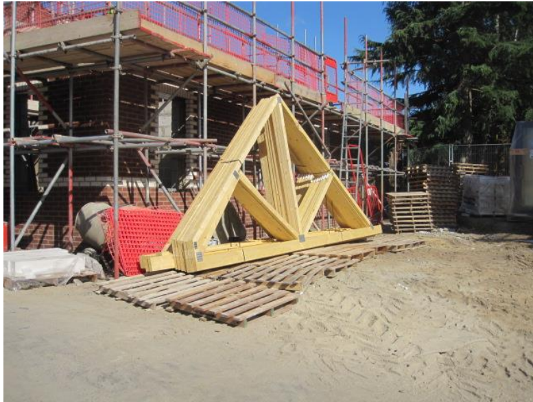
Roof trusses delivered for Parfitt
