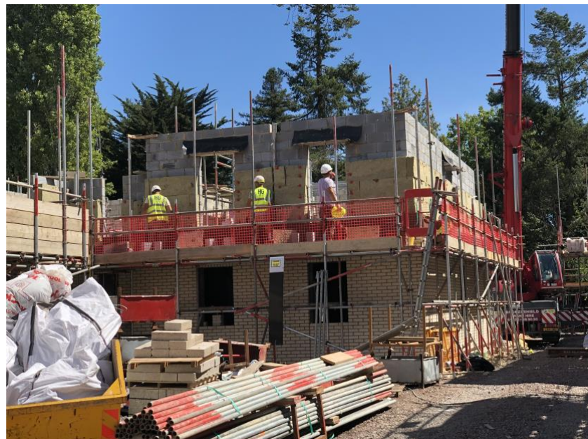
Brick and blockwork has continued on Townsend
