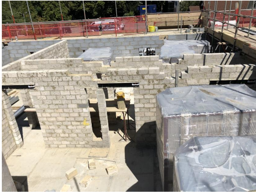
Looking into the 1 st floor rooms on Preedy
